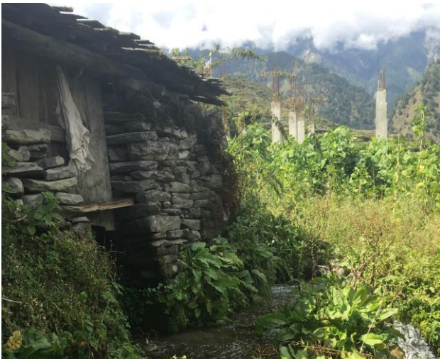
Figure 10. Downstream façade of a mill (Authors).
