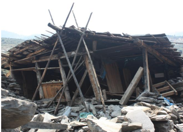
Figure 17. Collapsed house 2016 (Authors).
